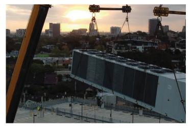
The four AHUs all incorporated EC fan motors for better efficiency. Having two chillers and four AHUs, provides the venue with greater flexibility for indoor comfort management. The system can be used at full capacity if race day operation requires all areas to be air conditioned, or it can be used in a banquet type mode to air condition certain hall spaces only outside of race days.
